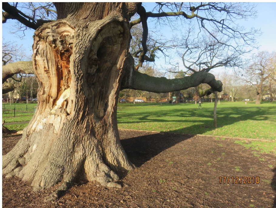
Photograph 6 The trunk of Bruce Castle Oak from the east. The two large branch wounds are decaying and wound-wood is forming around their margins. The left-hand wound was created around eight years ago and the right-hand one around 28 years ago. The low branch to the right is growing to the north and is propped 9.4m from its union with the trunk.
